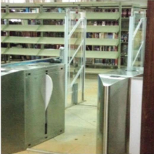
Photo 16: Electronic access control to enhance security at the library exit. This also ensures unauthorized IRs do not leave the library as this triggers the security alarm
