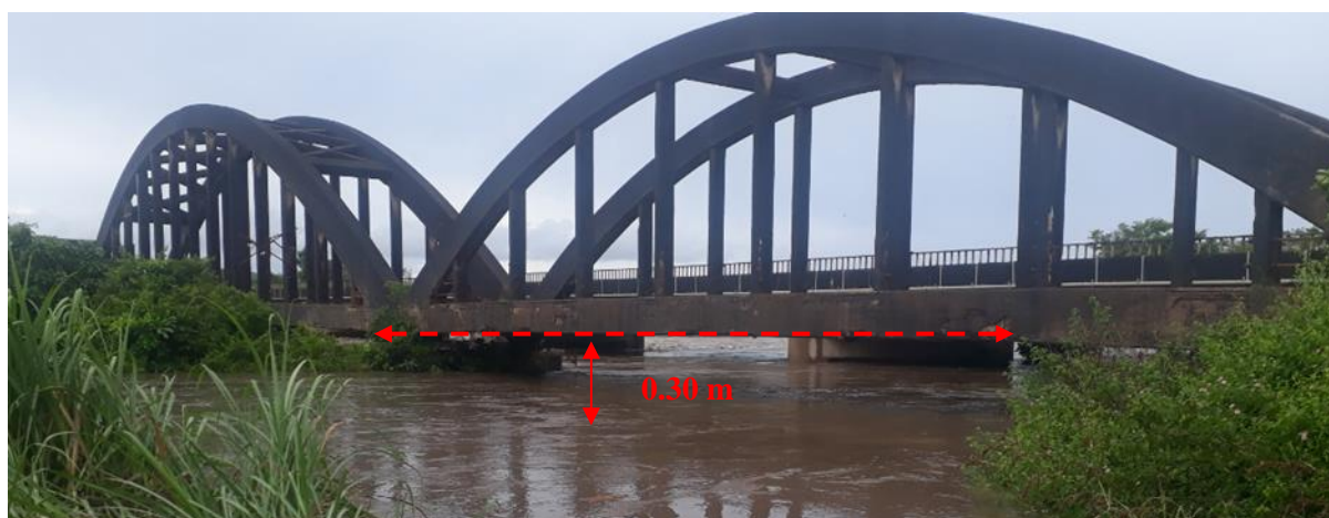
Photograph 3.14: Old Arch Bridge and R102 Concrete Bridge in the upper estuary during the May 2018 flood event several hours after the peak flood (Photo by Kelbe)
