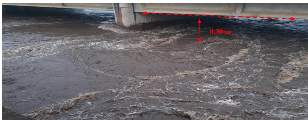
Photograph 3.15: Turbulent (super-critical) flow under R102 Road Bridge during the rising flood event in May 2018 (Photo by Kelbe)
