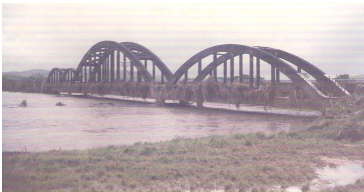
Photograph 5.1: The old N2 Road Bridge several hours later the main flood peak had receded following an approximate 1:100-year rainfall event in September 1987 (photo by Kelbe).
