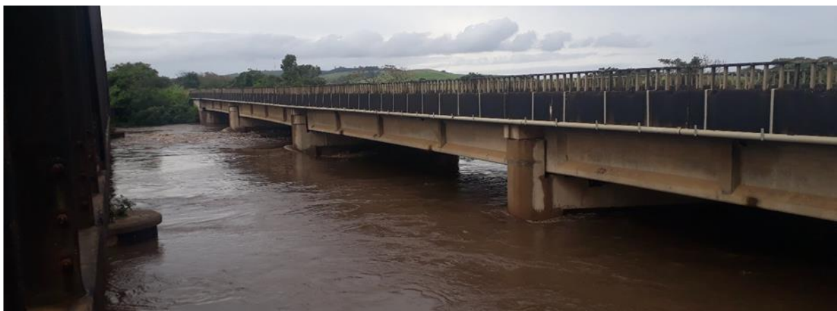
Photograph 3.9: The R102 Road Bridge (old N2 Bridge) in the upper estuary
