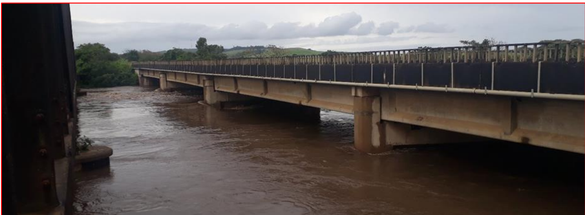
Figure 5.24: The simulated spatial extent of the flooding along the Mlalazi Estuary during a 1984 Imboa flood event. The photograph shows the May 2018 storm event's maximum peak level at the old N2 Road Bridge (photo by Kelbe).
