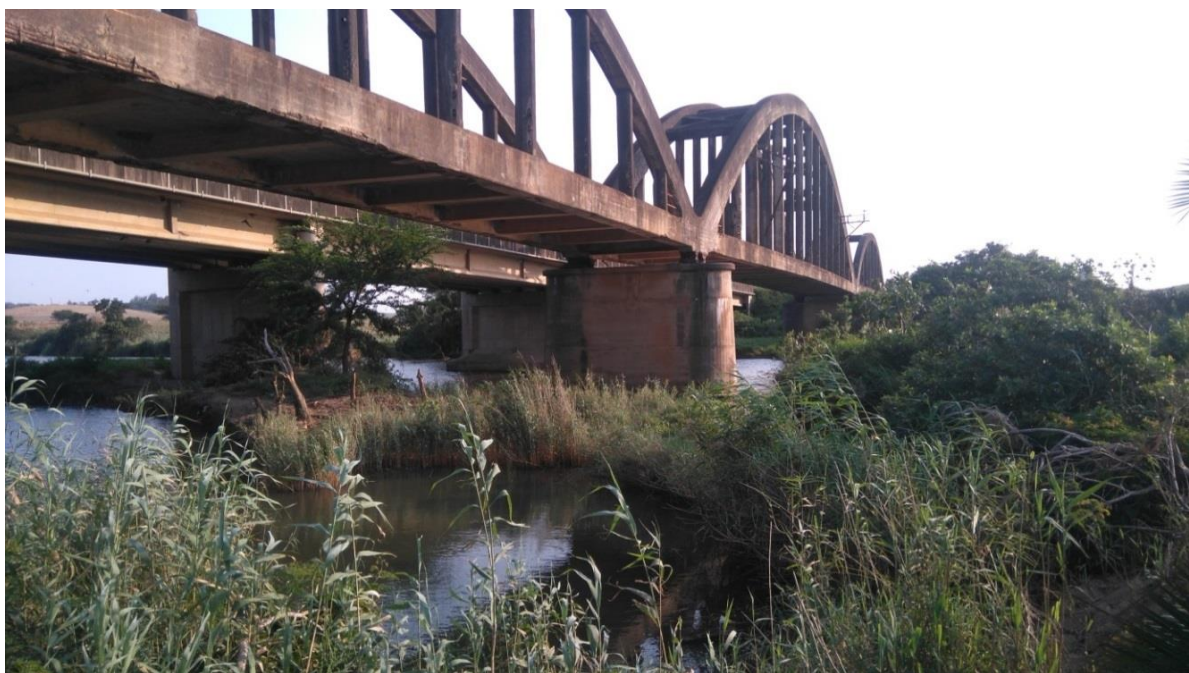
Photograph 3.10: The old arch bridge and R102 Road Bridge in the upper estuary
