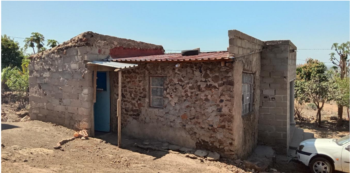
Figure 17: Tyre on the roof to self-protect from lightning. (Source fieldwork, September 2021)
