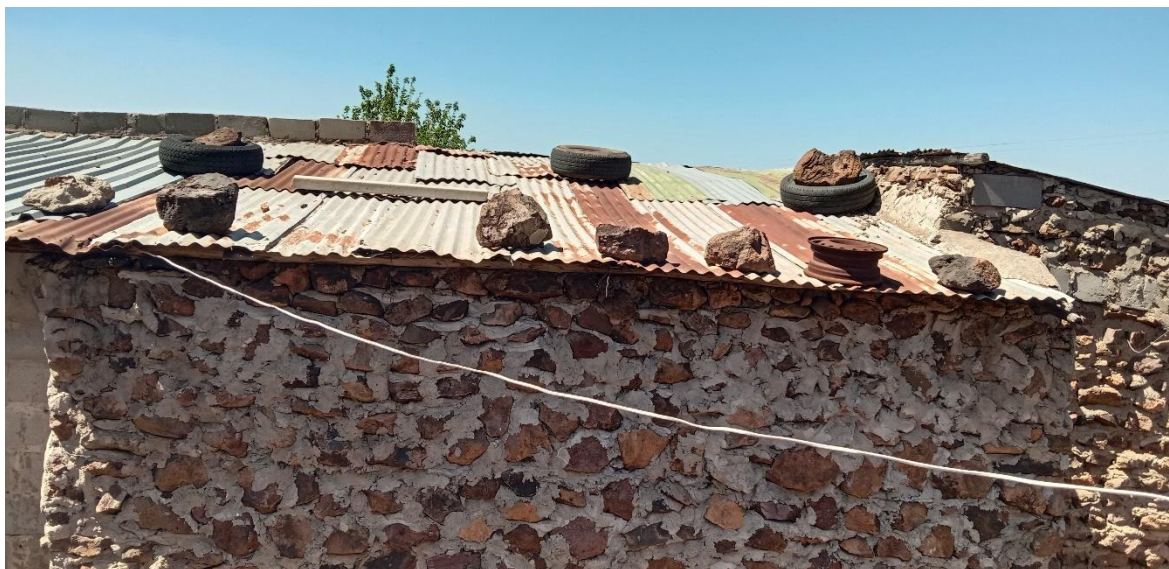
Figure 16: Tyre on the roof to protect from lightning (Source fieldwork, September 2021)
