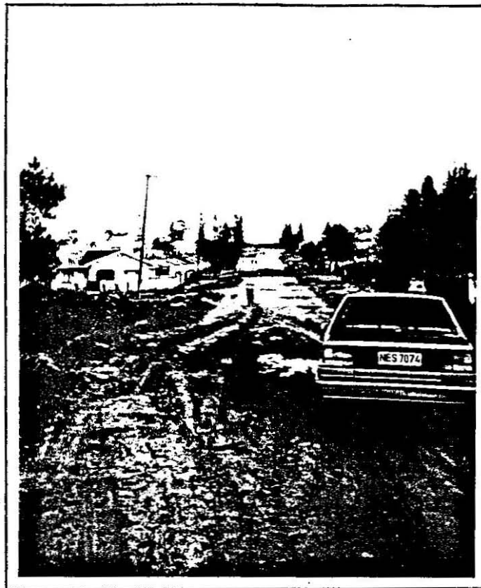
PLATE 23 : ROADS BADLY IN NEED OF REPAIR IN GEZINSILA
