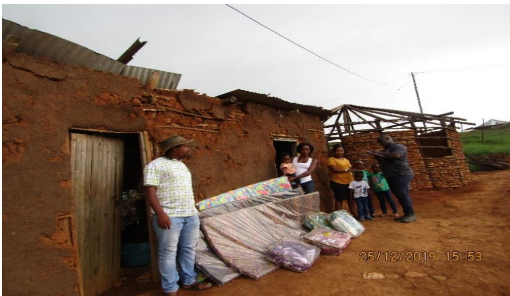
Figure 5.9: Houses made from iintingo (Source, Municipal Disaster Management Officer ubuhlebezwe local municipality, December 2019).
