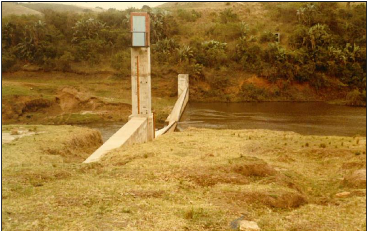
Figure 3.12: Gauging weir W1H012 on 16 January 1981 (DWS)
