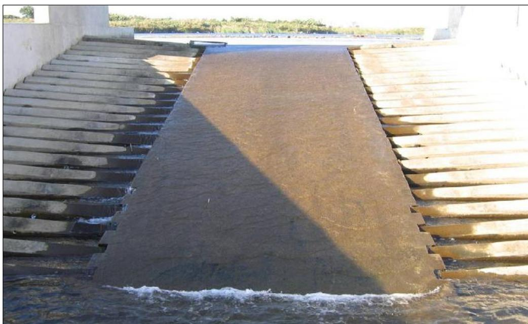
Figure 1.2: The Mzingazi gauging crump weir with the central spillway and double fishway showing the funnel trap at the fishway exit.
