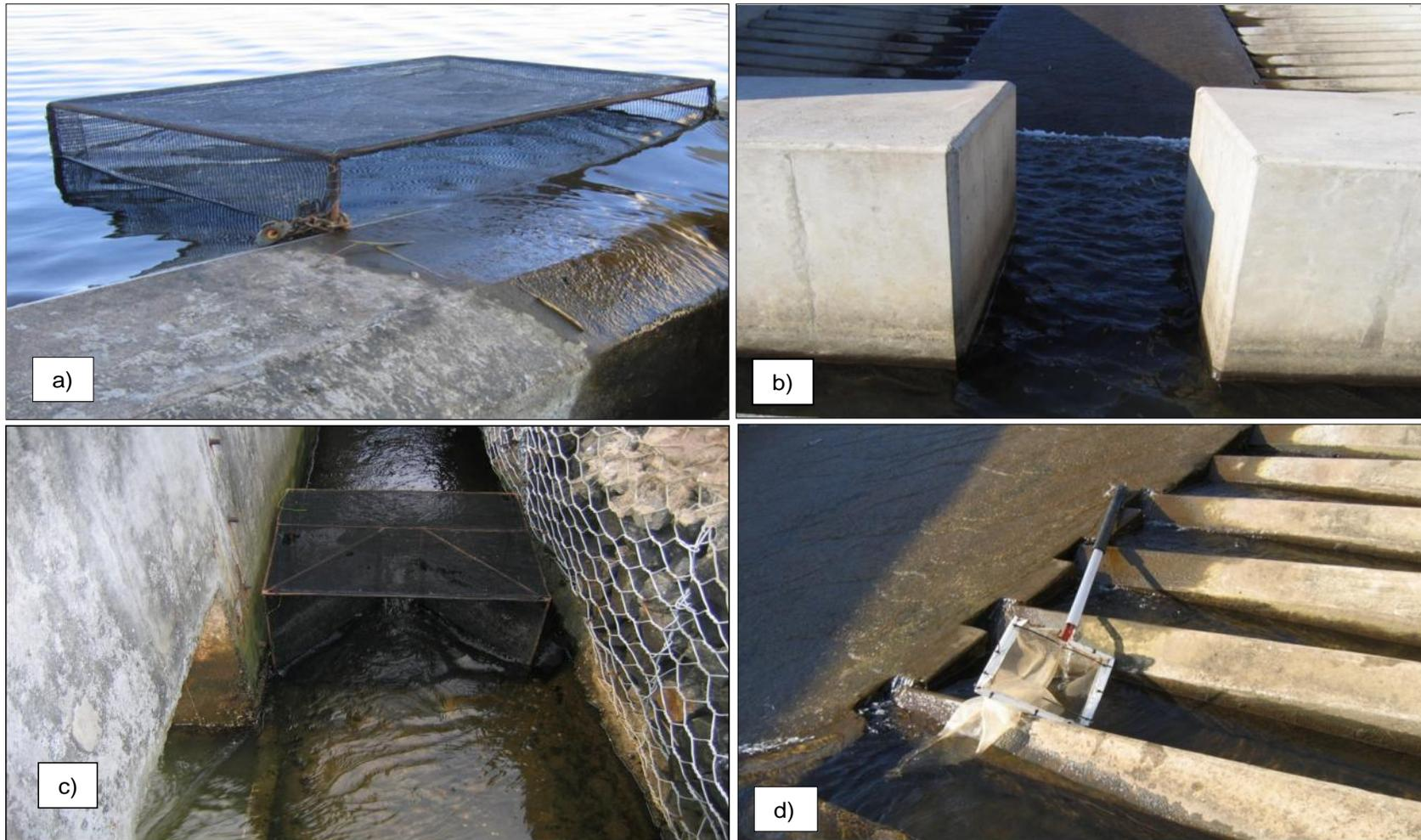
Figure 2.2: The Mzingazi fishway (a) exit and (b) entrance, the (c) Saltwater Barrier and (d) the Mzingazi fishway pools, showing the funnel traps and dip net used during the monitoring period.
