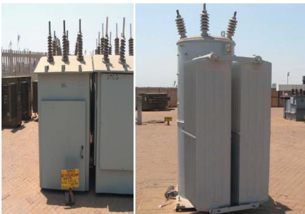
Figure A4.14: Kiosk (on the left) and Voltage Regulator (on the right)
