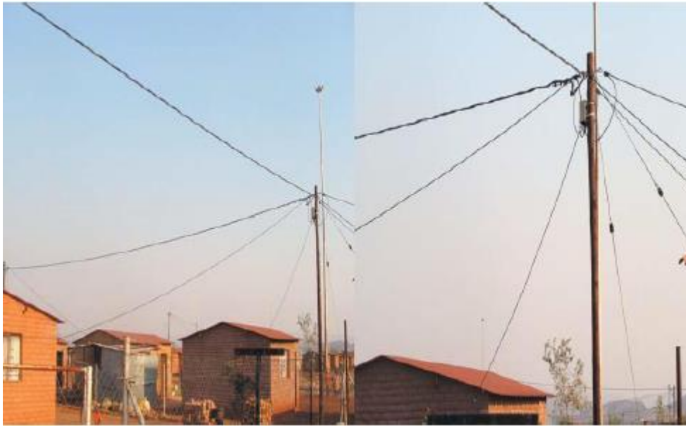
Figure A4.21: Various houses being electrified by means of airdac
