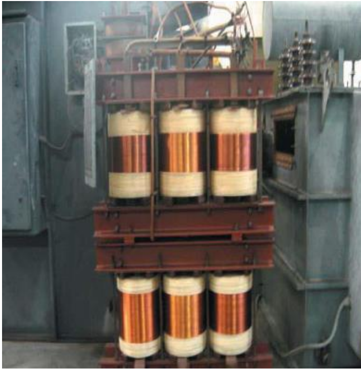
Figure A4.3: Inside of a transformer
