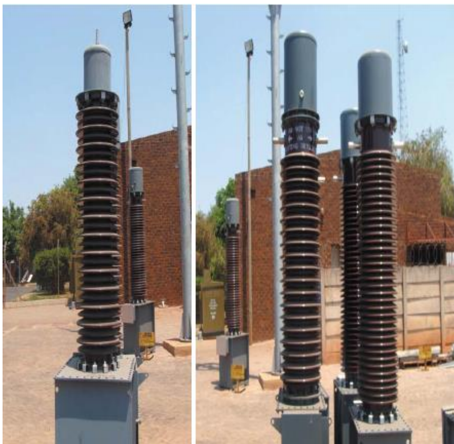
Figure A4.13: VT (on the left) and CT (on the right)
