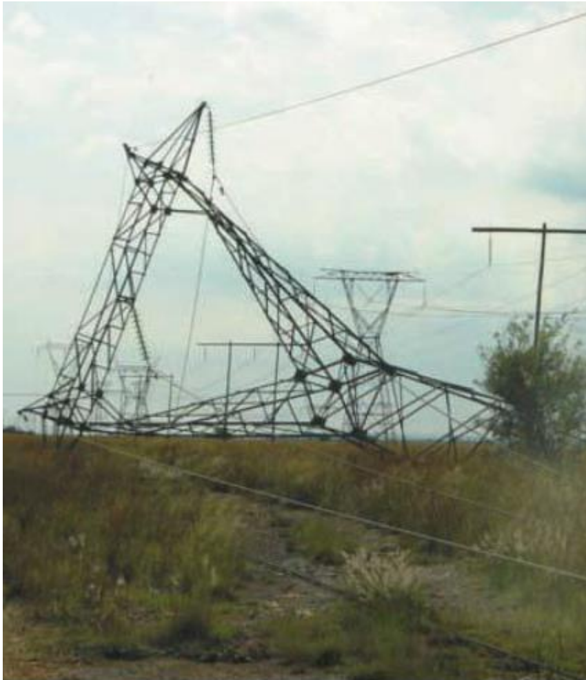
Figure A4.6: Collapsed Pylons
