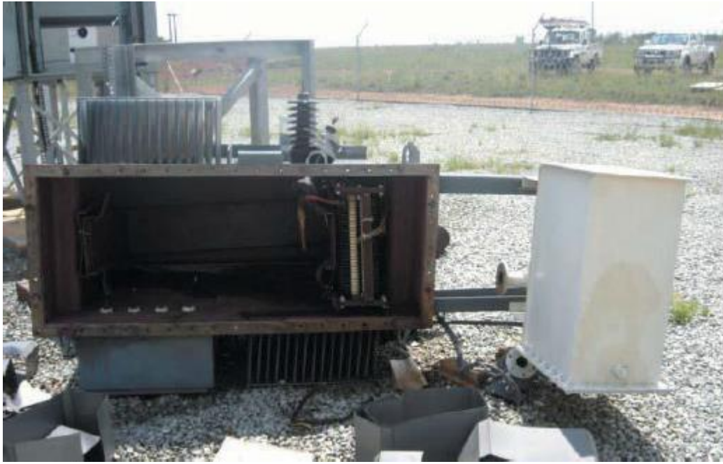
Figure A4.10: A substation transformer that was vandalised and the copper coils inside stolen.
