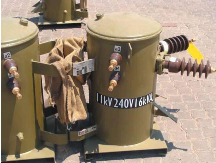
Figure A4.1: 11 kV Transformer
